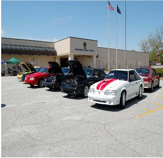
Spartanburg County Administration Building
