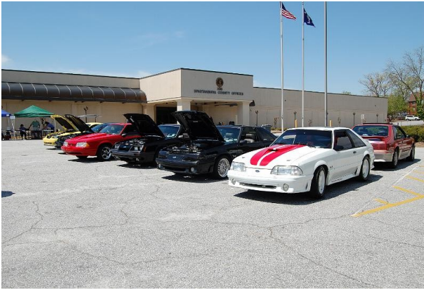
Spartanburg County Administration Building
